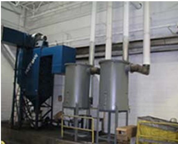
Weld and Fabrication Shop
