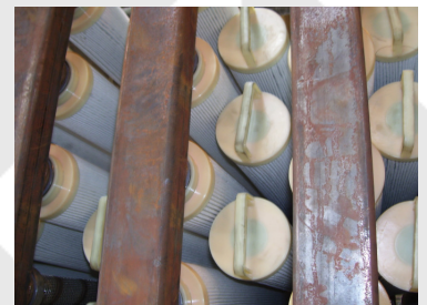
Compax coreless elements installed
