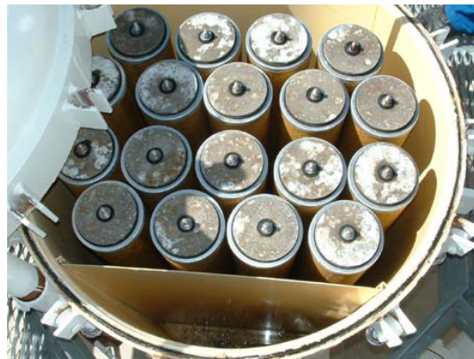
Figure 1 Typical 644 Filter Housing, showing installed elements. The threaded rod, “center-plate” and nut that is required to be tightened on the threaded center post is also visible.
