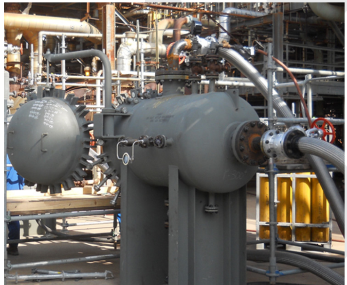
HRT rental vessel on location
